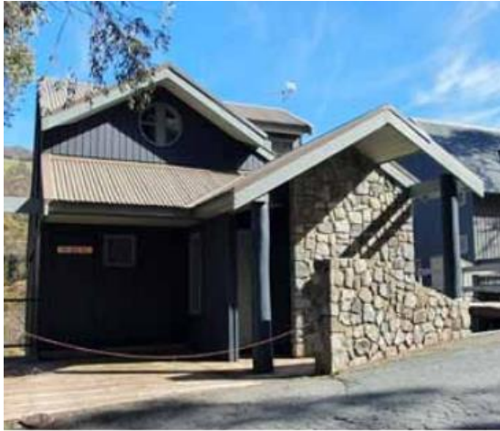
Figure 6: View of 2 storey detached lodge opposite the subject site
