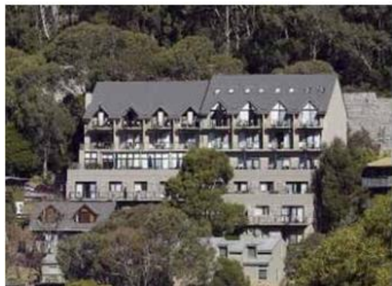
Figure 9: 'Lantern Apartments' tourist accommodation development located on Banjo Drive in the southern part of the Thredbo Resort
