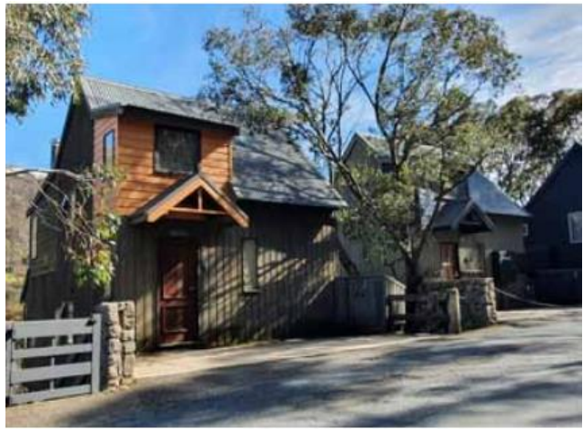
Figure 7: View of 2 storey detached lodge opposite the subject site
