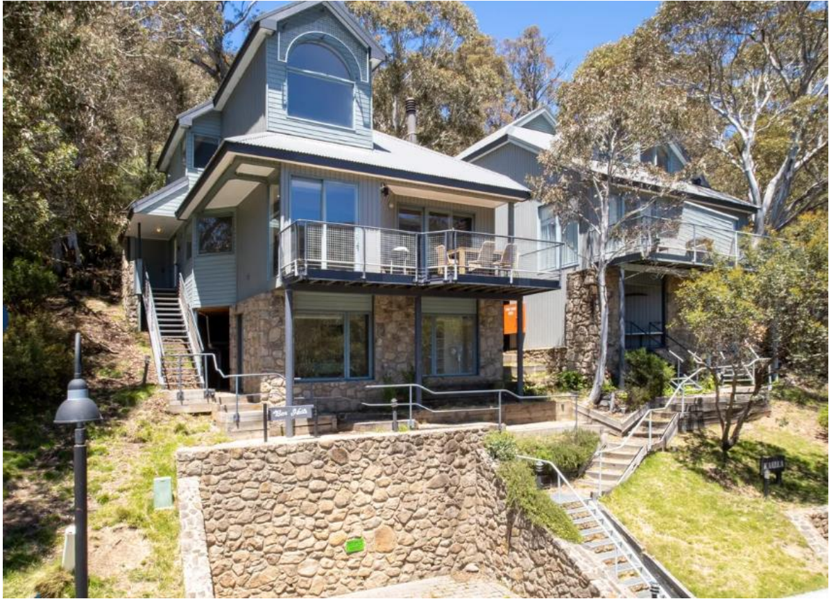
Figure 4: View of Ben Halls Chalet west of the subject site
