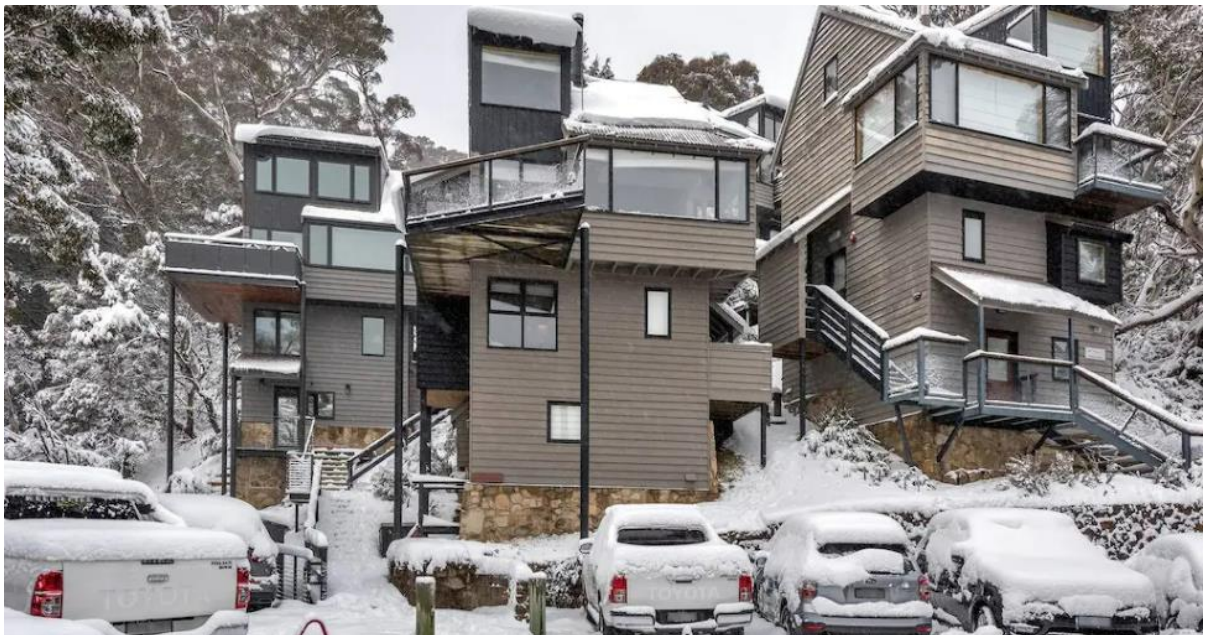
Figure 5: View of 3-storey detached lodges east of the subject site
