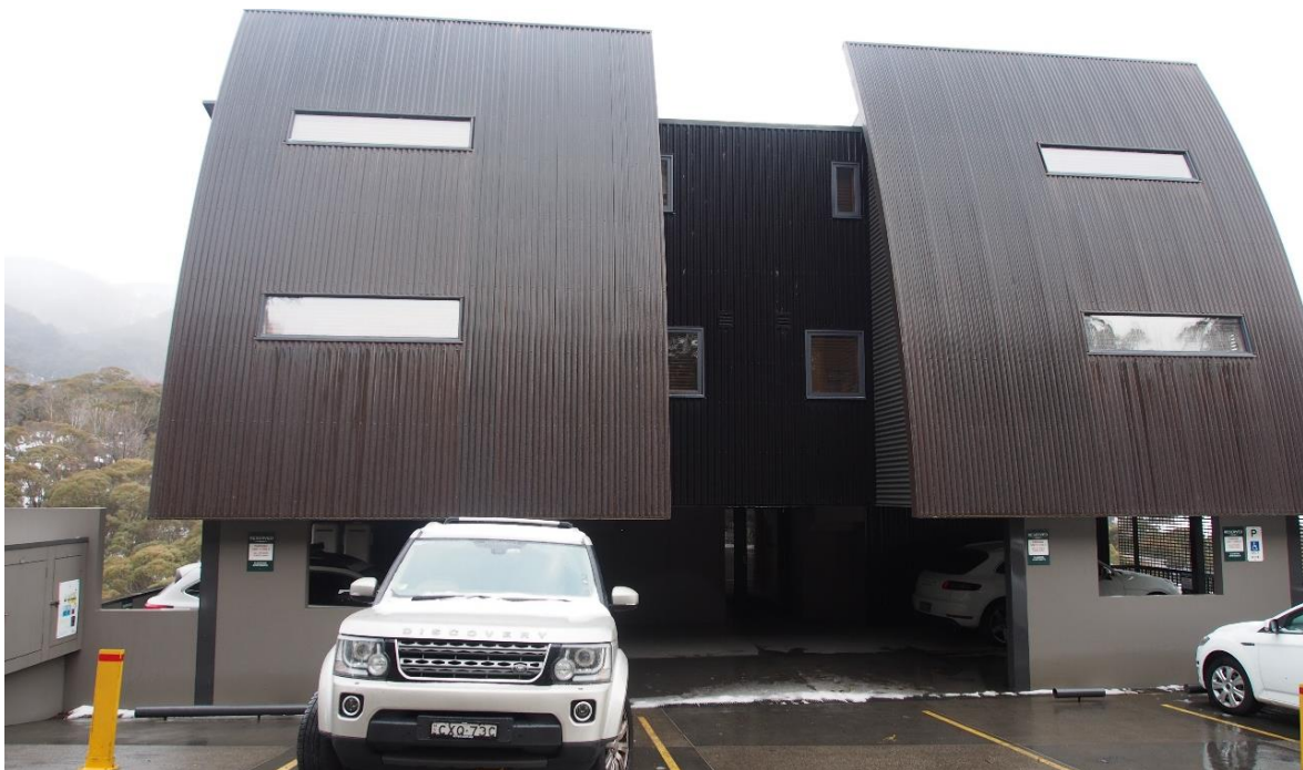
Figure 10: 'Elevation' tourist accommodation development located at 12 Bobuck Lane, Thredbo Village; view of Bobuck Lane building elevation
